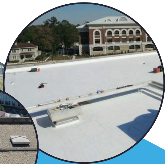
Valdosta Federal Courthouse | Valdosta, GA >> TPO Single-Ply Roof | 32,000 sq. ft.
